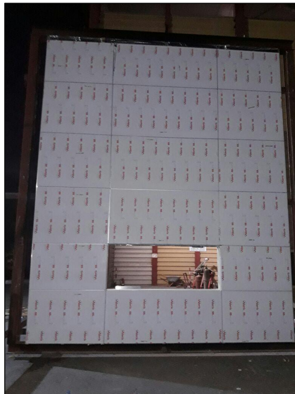
Picture 8: ALERIS aluminium panels after the installation.
