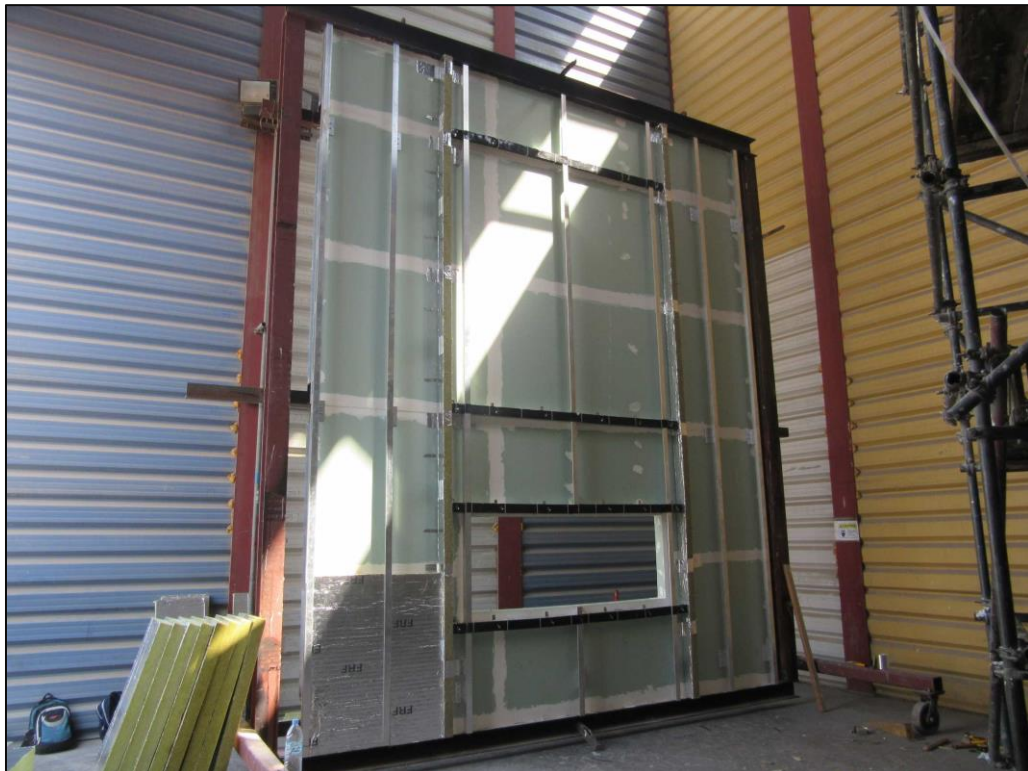
Picture 4: Elevation showing the SIDERISE RV/RH fire barrier system after installation.
