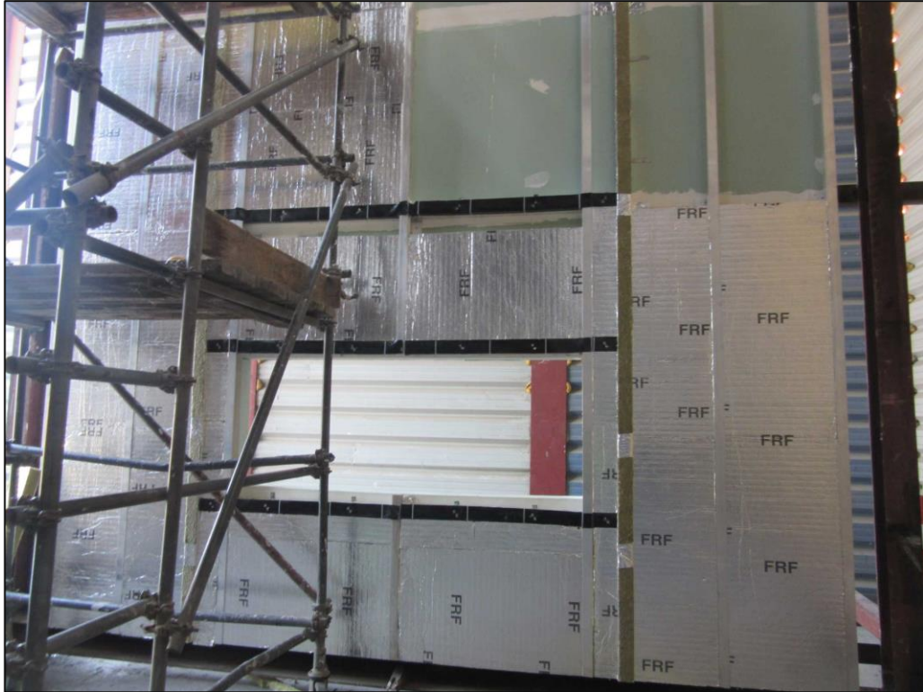
Picture 5: Mineral wool insulation slabs fixed onto the base wall.
