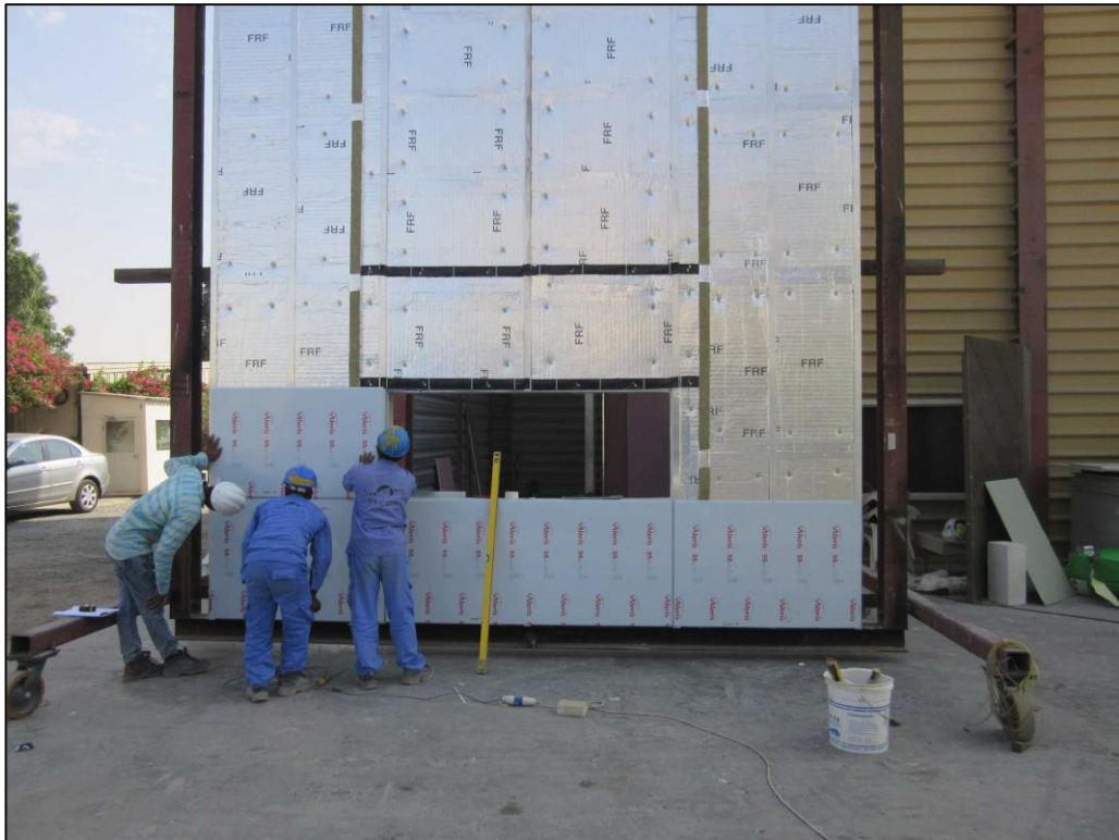
Picture 7: ALERIS aluminium panels being fixed onto the runners.
