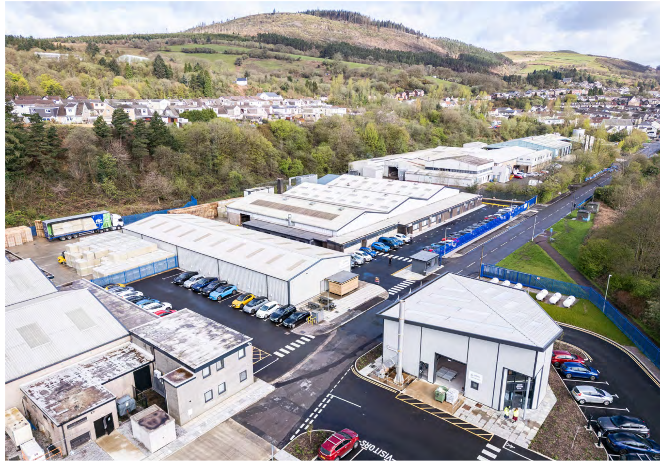
Siderise Insulation manufacturing facility and Global Innovation Centre in South Wales
